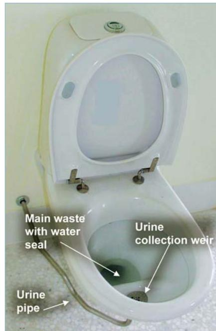
**Figure 1. The wall mounted Gustavberg urine separating toilet at an Ecovillage home showing the urine weir at the front of the pan, urine collection pipe and the main waste with the water seal.**
