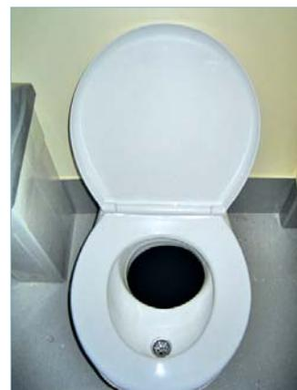
Figure 3. Urine-separating dry toilet pedestal.
